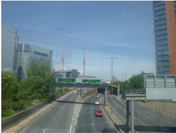
Figure 3: Existing photo from pedestrian bridge over East India Dock Road/Aspen Way
