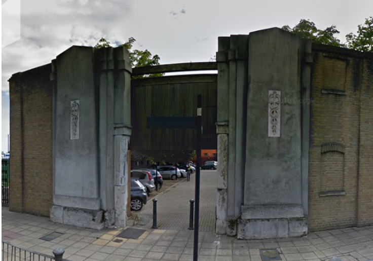
Image showing Grade II listed Entrance Gateway
